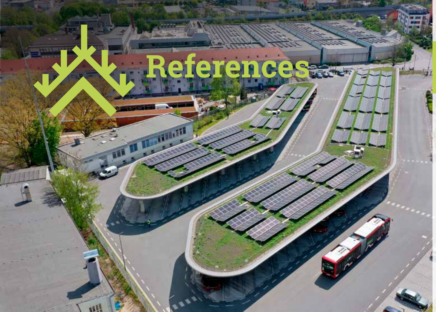
eBus Port, Nuremberg Extensive green roof with solar system
