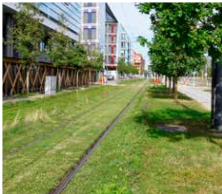
Planting track greening with grass
